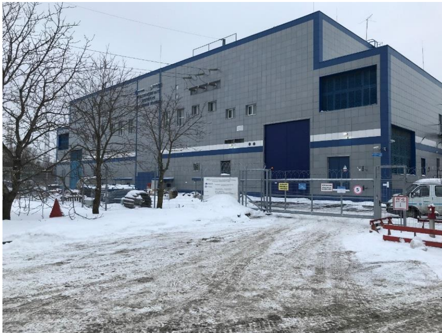
Renovation of Substation No. 18 Krasny Treugolnik converted to 110 kV
